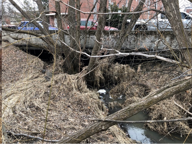
FIGURE 1.3: BOX CULVERT OUTLET
