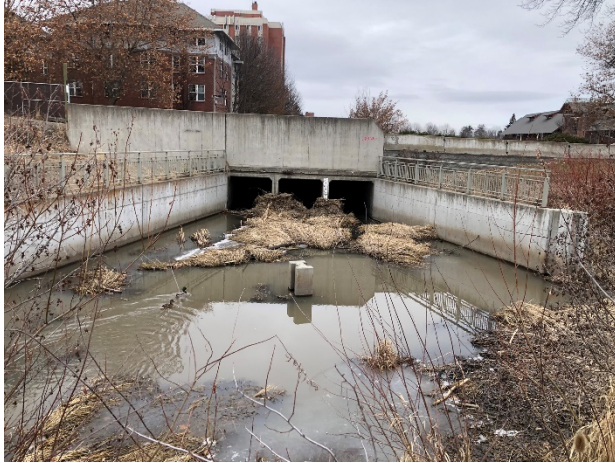
FIGURE 1.2: BOX CULVERT INLET
