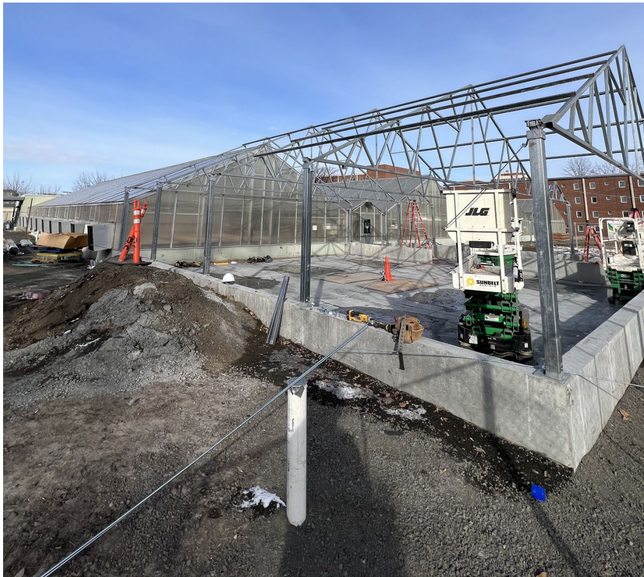
Figure 1 Erection of greenhouse
