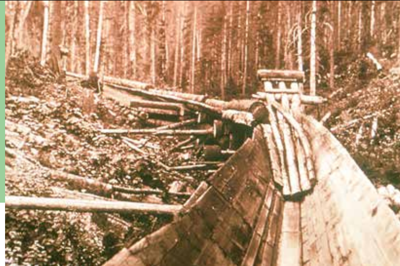
Logs being moved downhill in a flume.
