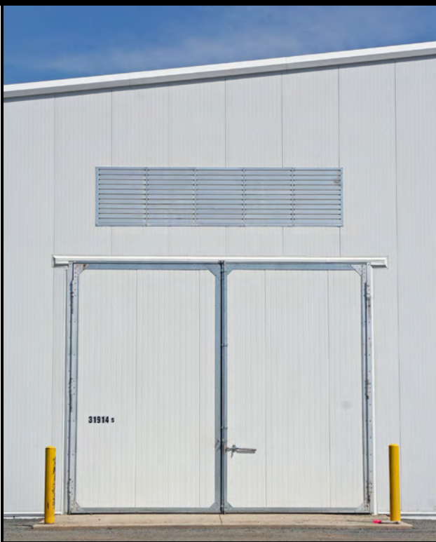
Figure 2.9. Exhaust louvers above access doors.
