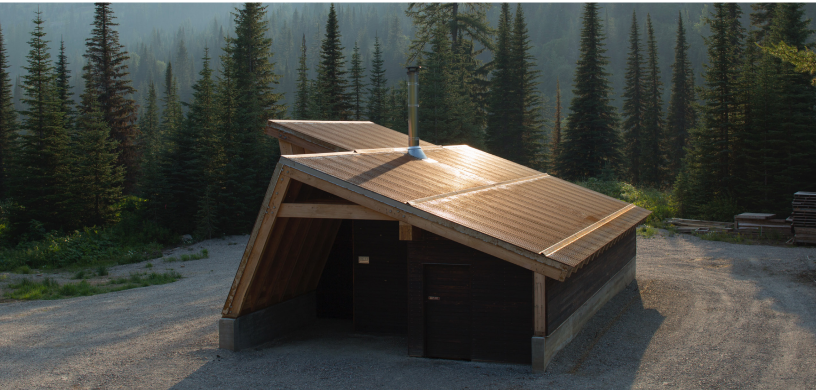
Snowmobile warming hut. Designed and build by UI architecture students for the US Forest Service north of Sandpoint, ID.
