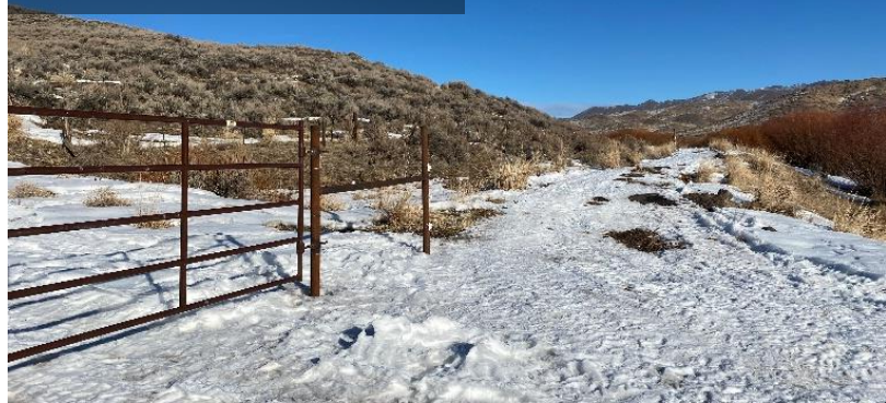
METAL H-BRACE AND GATE
